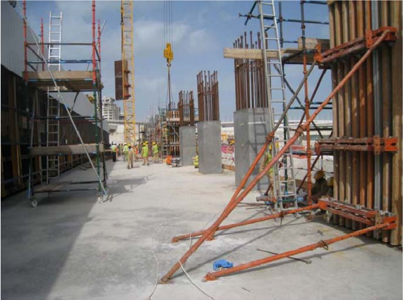
Tower 1- Construction of columns in progress
