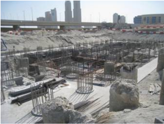
Tower 4-Installation of jump form shutter in progress.
