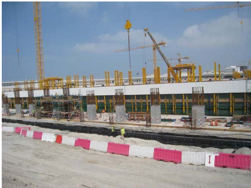
Construction of columns in progress
