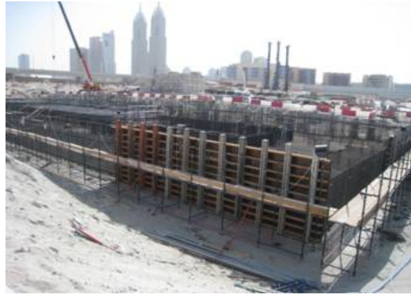
Tower 3- Construction of column and reinforcement.
