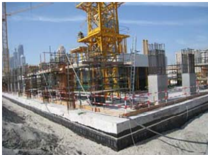
Tower 3- Construction of columns in progress.
