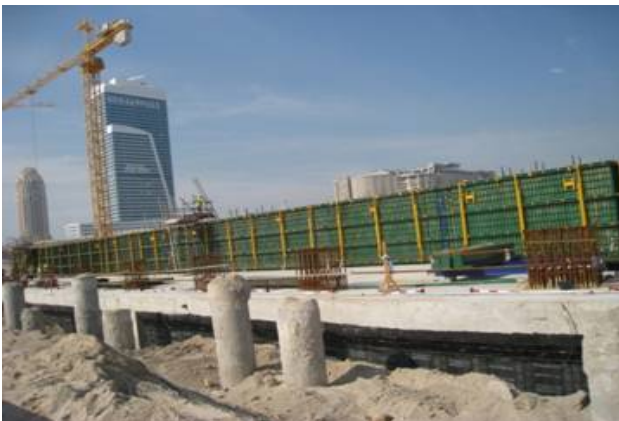
Installation of jump form shutter completed
